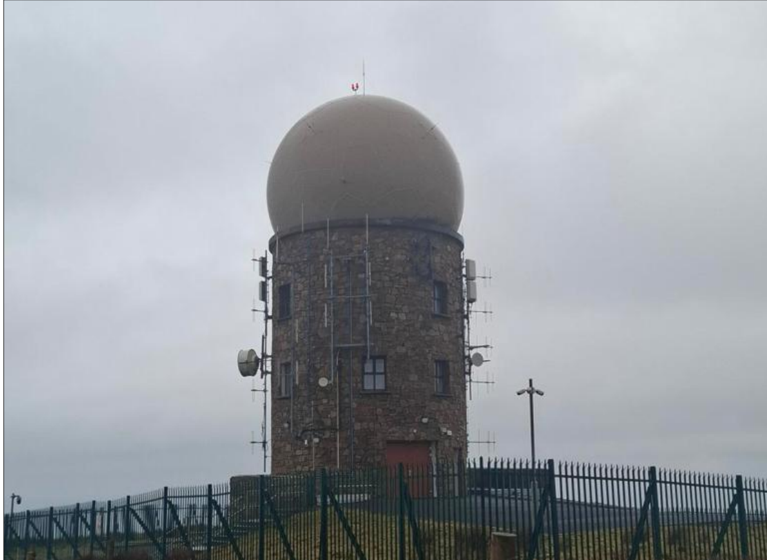
Figure 11. Dooncarton Radar Station
